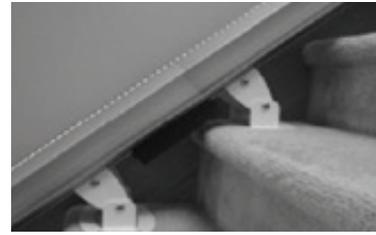
**Step 11:** The underside of the rail must be at least 2" above the stair tread nose to provide clearance for the footrest. **To achieve this 2" clearance move the rail and bracket forward.** Once the clearance is 2" tighten all bracket nuts to hold the brackets in position. To maintain the 2" clearance, and to hold the rail in place, secure the bottom bracket to the first step from the floor with 2-2" wood screws, using a  $\frac{3}{8}$ " nut driver on a 6-10" extension of a cordless drill.
