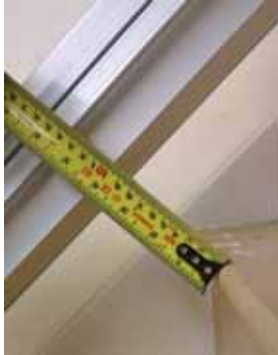
RAIL TO STEP NOSE MINIMUM OF 3 1/4"
