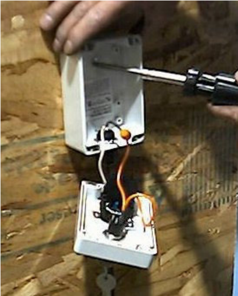
FIG. 17- MOUNT LOWER CALL STATION
