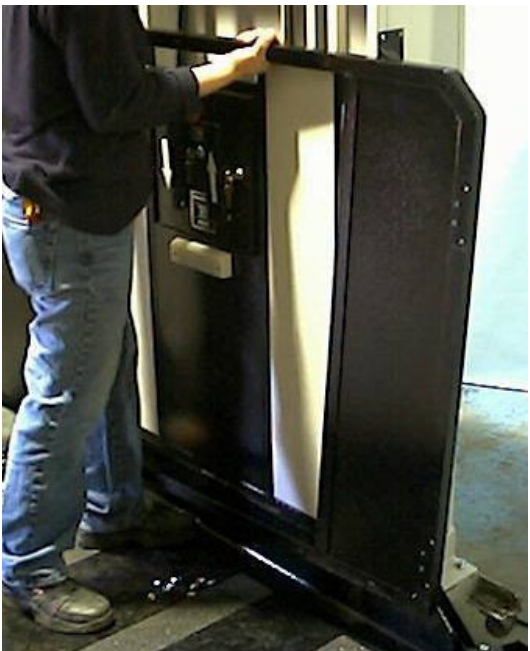
FIG. 5A- INSTALLING CONTROL WALL EXTENSION
