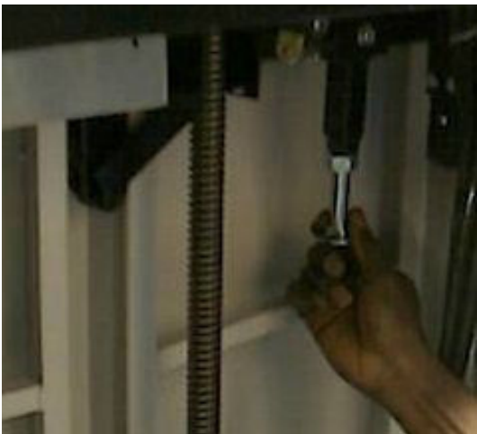
FIG. 4- INSTALLING LOWER MECHANICAL STOPS
