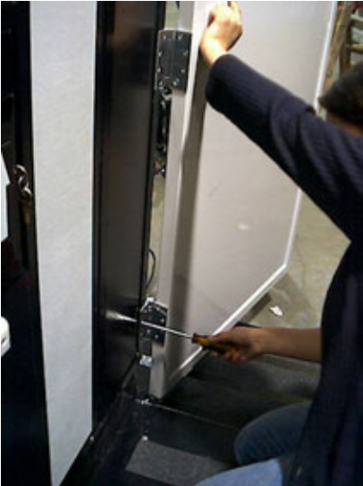
FIG. 8- MOUNTING GATE TO CONTROL WALL EXTENSION
